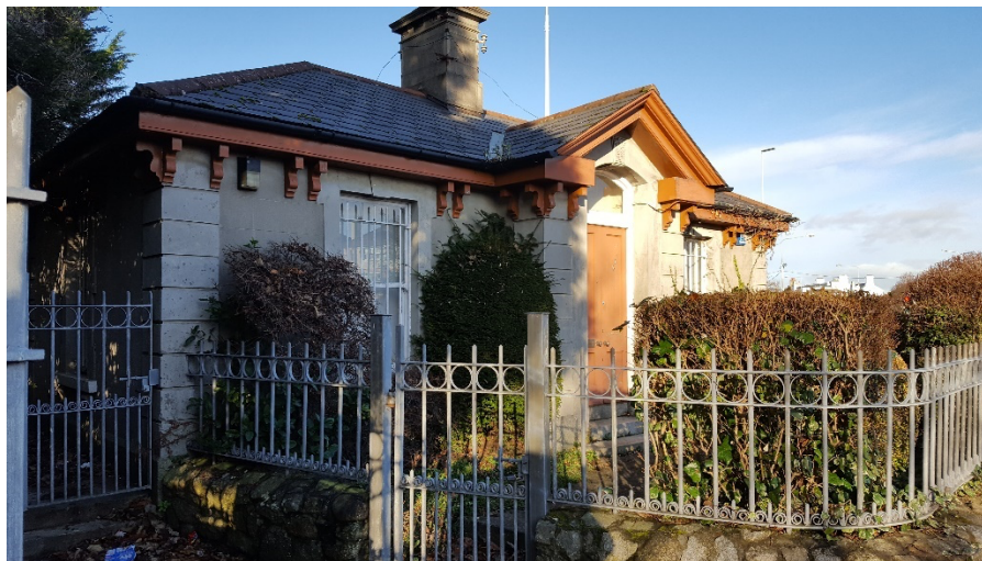
Lodge at St Teresa's House
